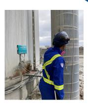
We also offer complete thermal energy measurements that can help you evaluate the performance of your heat exchangers or the proper operation of your cooling towers. Our RTD clamp on temperature sensors, which are matched and paired, offer an accuracy of 0.06°C.
